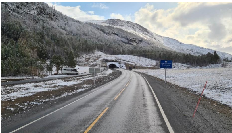
Picture above: a tunnel towards the NO-SE border on the way back
